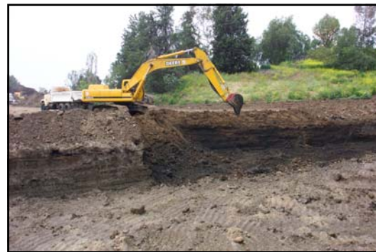
Excavation of Former Oilfield Sump
